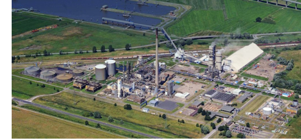
Urea plant of Yara at Brunsbüttel (Germany)
