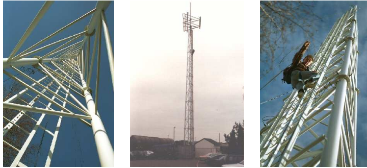
Figure 4.4: Vibration measurements on a steel transmitter mast were used to evaluate the performance of the algorithm proposed in this chapter. The transmitter mast is located in Antwerp, Belgium and is part of a cellular phone network.
