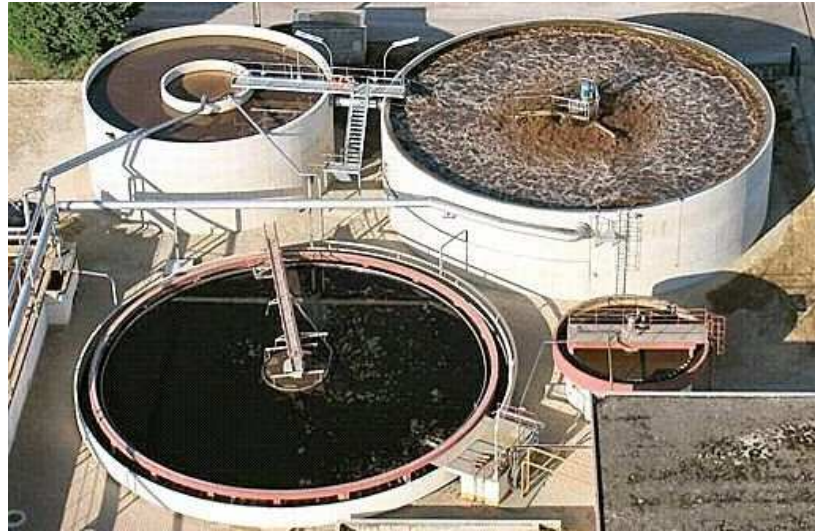
Figure 4.3. Detection of a leak in a waste water treatment process (from Rao [146]). Top: Illustration of the connected tanks process. Bottom: Aerial photograph of a typical waste water treatment plant.
